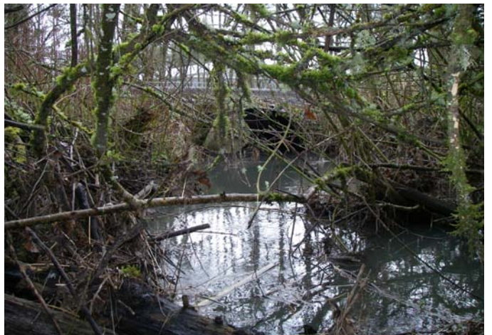
Unit 58 - End of survey at culvert crossing and Harding Road.
