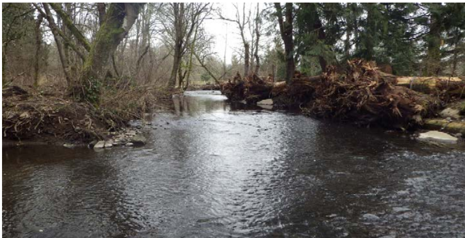
Unit 4 - looking upstream at log habitat structures
