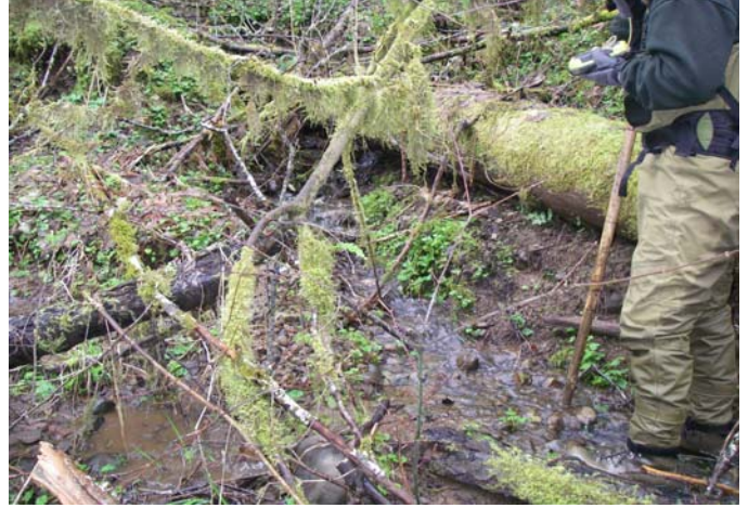
Unit 1 - Small tributary with large wood placement.
