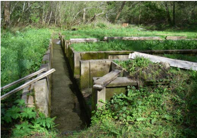
Raceways at Brush Creek Hatchery.
