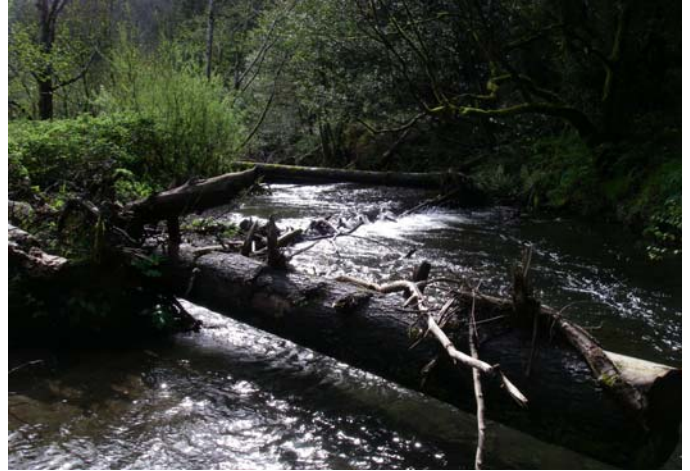
Upstream view of large wood placements for habitat structures.
