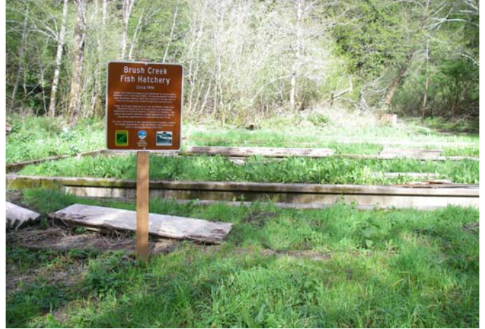
Partially deconstructed Brush Creek Hatchery.
