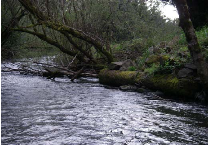
Downstream view of roadside bank stabilization.
