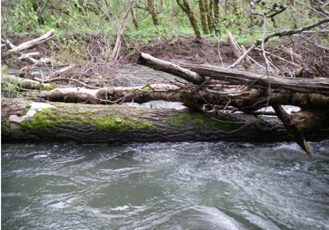
Upstream view of placed large wood accumulating debris. Near start of survey.
