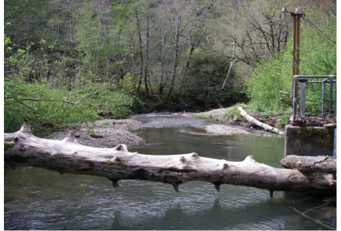
Downstream view of placed large wood habitat structure.
