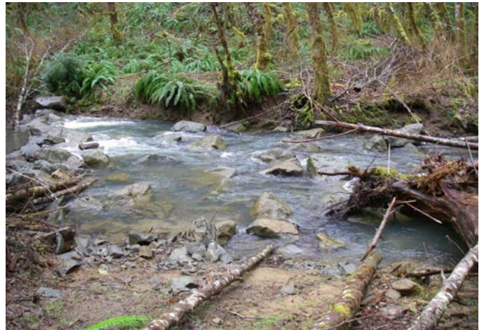
Placed boulders and large wood for habitat structures.
