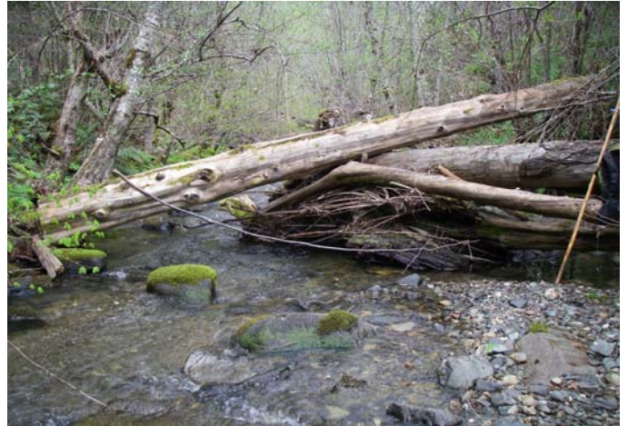
Unit 15 - Downstream view of placed large wood structure.
