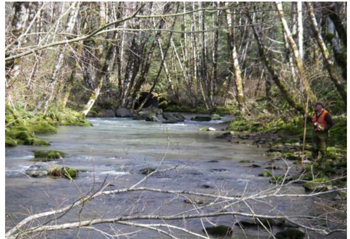
Upstream view of confluence with North Fork Big Tom Folley Creek. North Fork Big Tom Folley Creek culvert in background.
