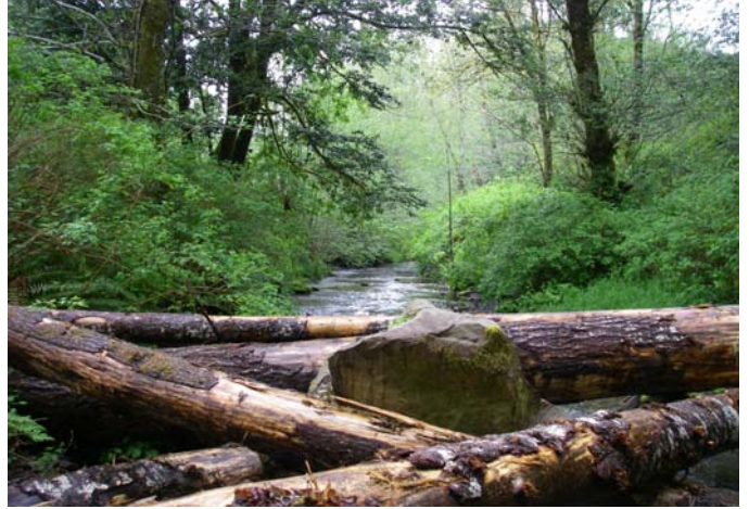
Upstream view of large wood and boulder placement for habitat structure.
