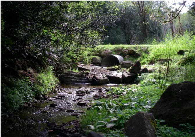
Upstream view of culvert and road crossing upstream from start.
