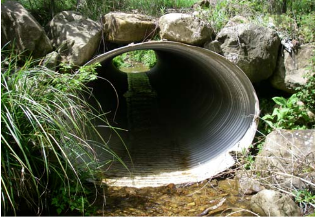
Downstream view of culvert near the end of the survey.
