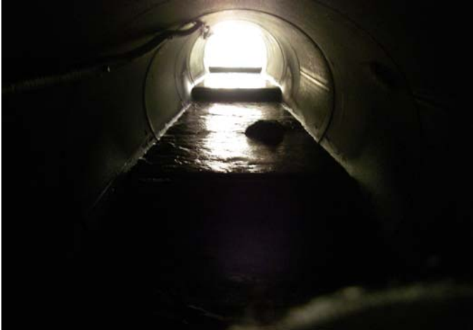
Unit 1 - Upstream view of Hwy. 101 culvert at start of survey. Hwy. 101 crosses here.
