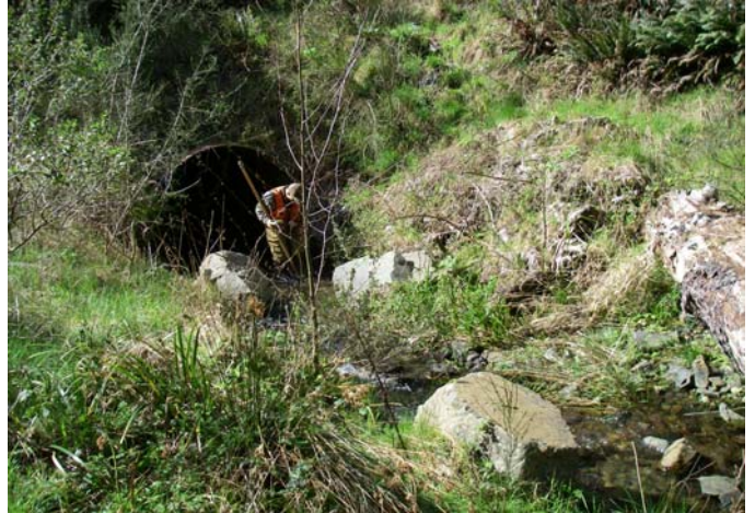
Unit 2 - Downstream view of upstream end of Hwy. 101 culvert.
