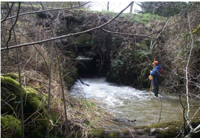
Culvert crossing at unit 26. Nick Chambers in photo.
