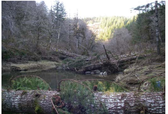
Unit 2 - Large wood placement.
