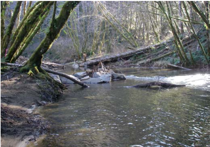
Upstream view of boulder and large wood placement.
