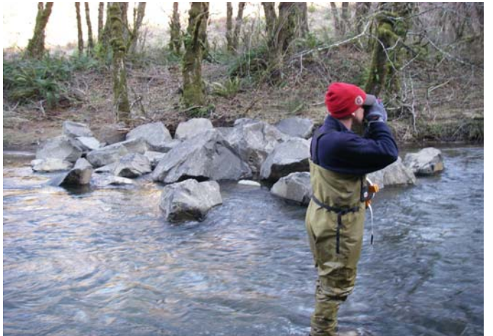
Placed boulders for habitat structure.
