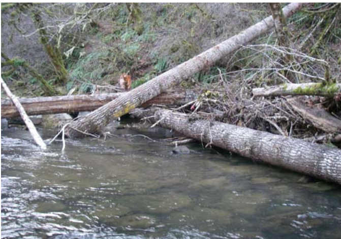
Large wood and boulder placement.
