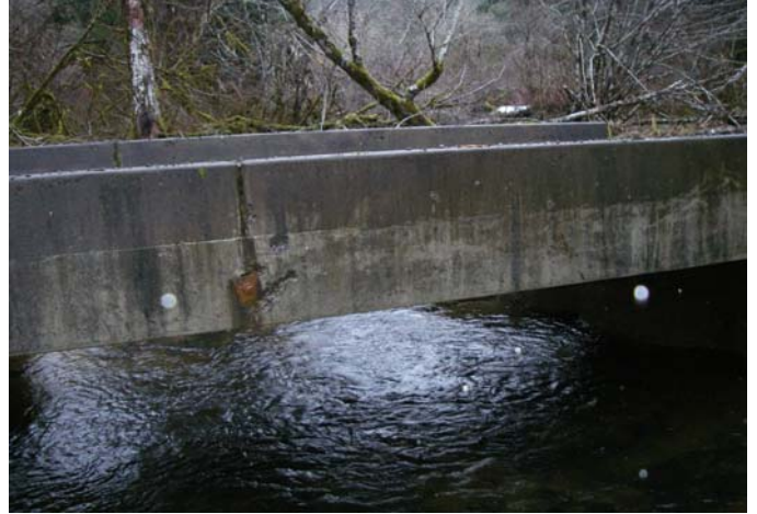
Unit 1 - Looking downstream from the survey start at bridge crossing.
