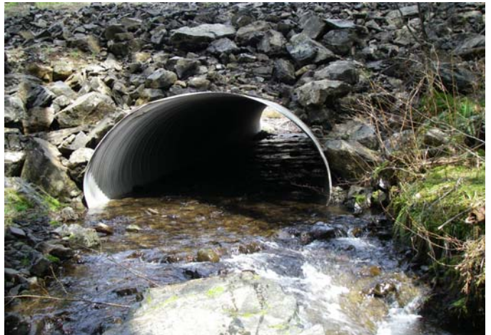
Unit 42 - Culvert crossing at Cruiser Creek Rd.
