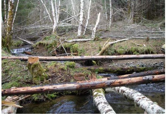
Unit 20 - Upstream view of large wood placement. Limited view of a right bank tributary confluence.
