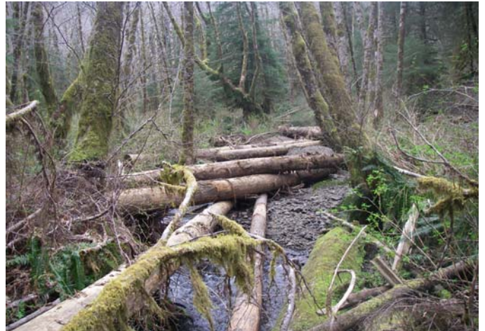
Unit 75 - A upstream view of the riparian area and large wood placement.
