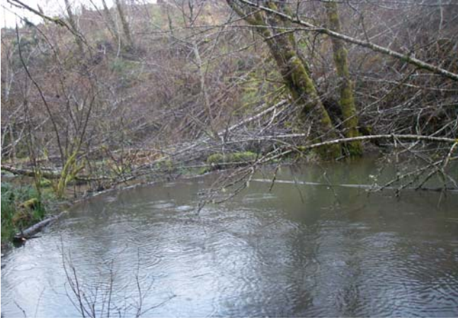
Unit 118 - Downstream view of beaver dam and pool.
