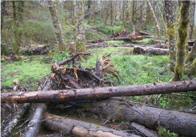
Unit 20 - Large wood placement within active channel and terrace.
