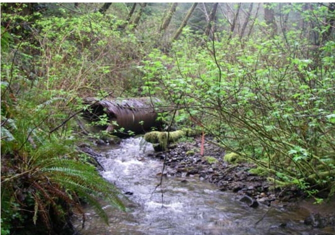
Un-used culvert near mid-point of survey.
